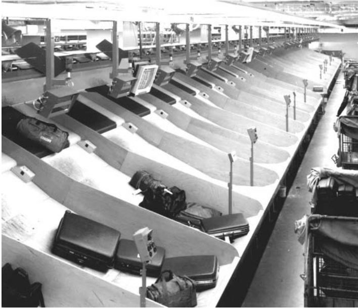
Figure 4.27. Terminals: chutes [Photo: BEUMER]
